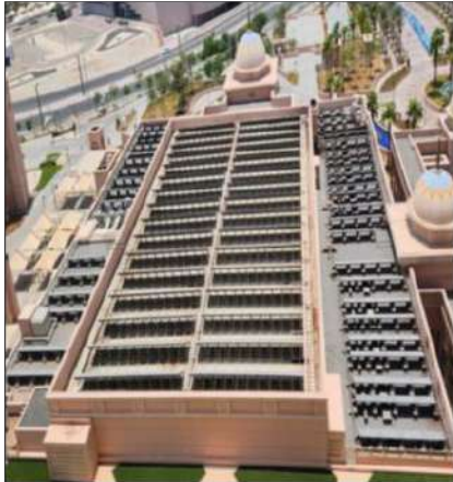
Solar panel in building roof for Heating boiler
